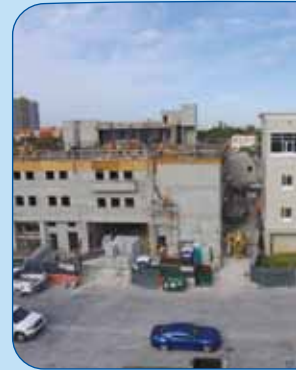
WEEK OF MARCH 20, 2017: Partially completed Miami Lighthouse Learning Center for Children™ is on the left
